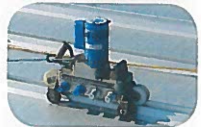
Butler's exclusive Roof Runner ® completes the industry's only field-formed 360-degree Pittsburgh double-lock seam.
